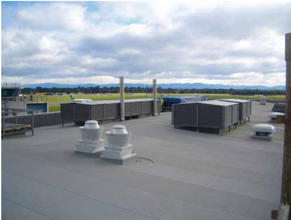
The new Christchurch Airport Terminal has been covered with 1.5mm Dove Grey Butynol.
